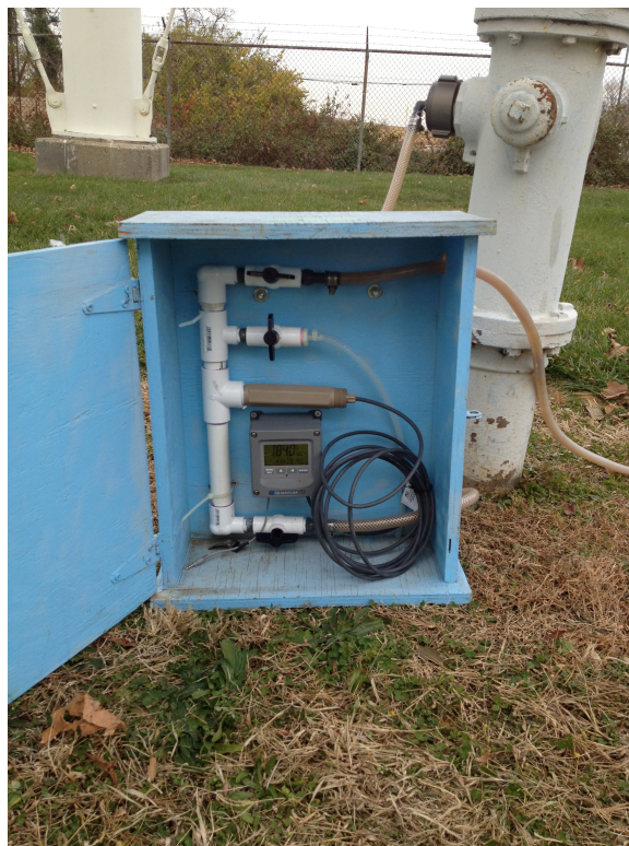
Figure 3: Continuous conductivity analyzer components (typical).
